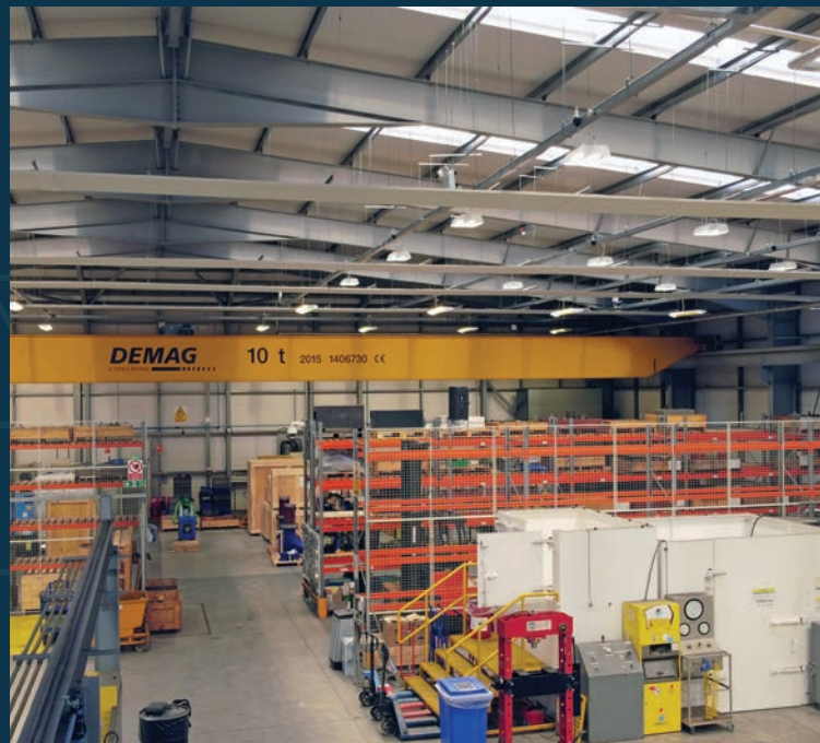
10 TONNE OVERHEAD CRANE VIEW FROM MEZZANINE
